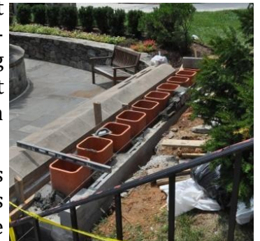
new wall with completed niches before capstones are placed
